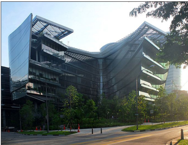
LucasFilm's Sandcrawler building in Singapore uses Solarban 72 glass containing a triple-layer of silver.
